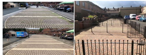
Cleaning of Car Park Areas
